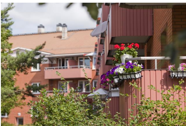
Rikshem's property Svärdslijan in Gideonsberg, Västerås, was built in the 1950s and renovated in the mid-1980s. The 254 flats in the area all have a balcony.
